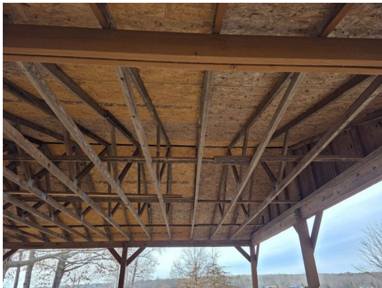
Underside of picnic shelter roof — OSB decking and rafters/trusses (Item #11)
