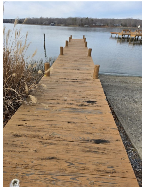
Boat launch dock walkway, with the newly-replaced multi-finger main slip dock visible beyond (Items #15-#16)
