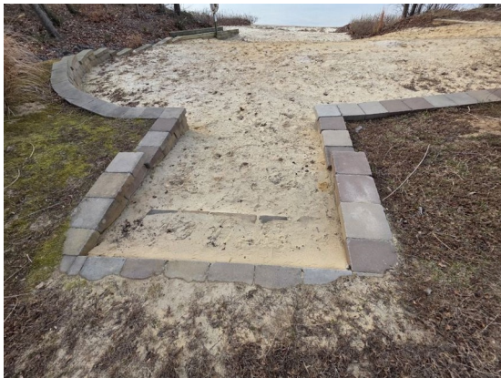
Sand beach access with paver edging — note pavers now in place of the 2010 wood timber retaining wall (Item #20, formerly Item #8)
