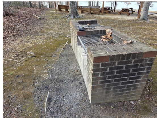
Brick masonry grill, alternate view
