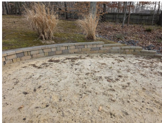
Sand beach and paver retaining wall, close view
