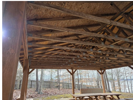
Underside of picnic shelter roof, alternate bay, showing truss plate connectors (Item #11-#12)
