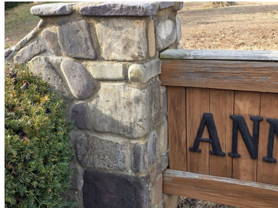
West entrance monument, corner detail with coursed stonework (Item #1)
