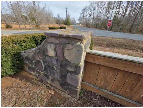
Monument pier corner detail, coursed stonework (Item #1)
