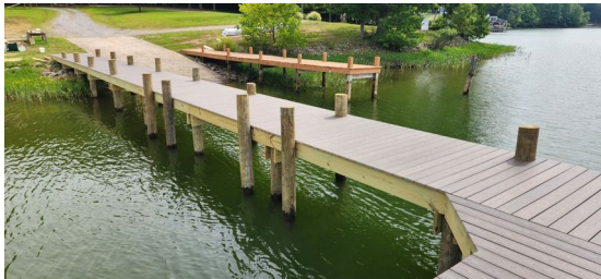
New main slip dock, elevated view down the center walkway (Items #15-#16)
