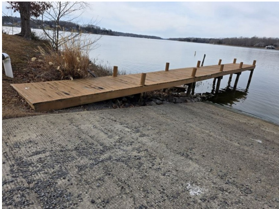
Boat launch dock and concrete boat ramp, prior to the approved repair (Items #17-#19)
