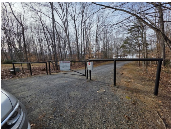
Metal pipe-rail entrance gate at the recreation area, open (Item #6)
