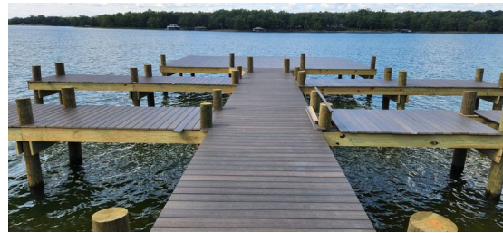
New main slip dock, straight-on view down the center walkway with finger slips on both sides (Items #15-#16)
