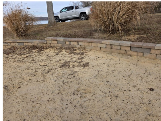
Paver retaining wall along sand beach, alternate view
