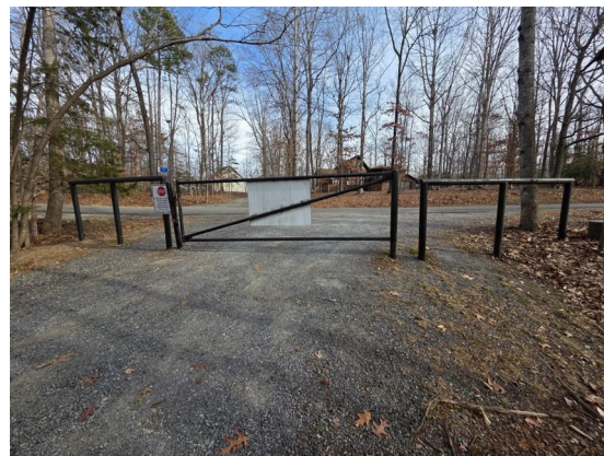
Metal pipe-rail entrance gate, closed (Item #6)
