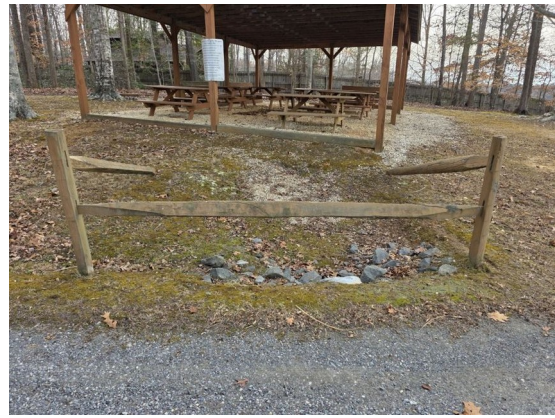
Split rail fence near the picnic shelter — appears in sound condition (Item #7)
