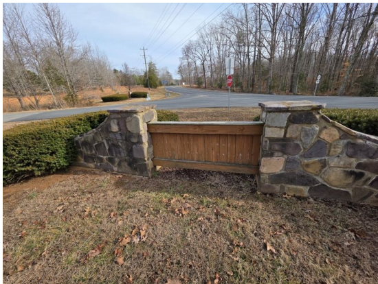
Wood-panel infill between stone piers, overall view (Item #2)
