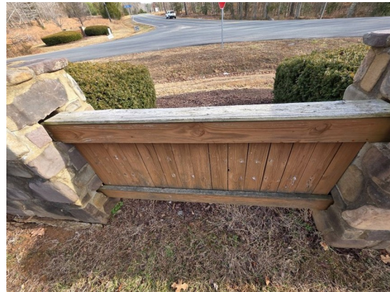
Wood-panel infill, close view — weathering and surface staining visible (Item #2)
