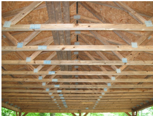
View of wood trusses
