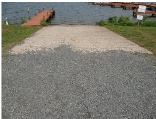
View of concrete boat ramp
