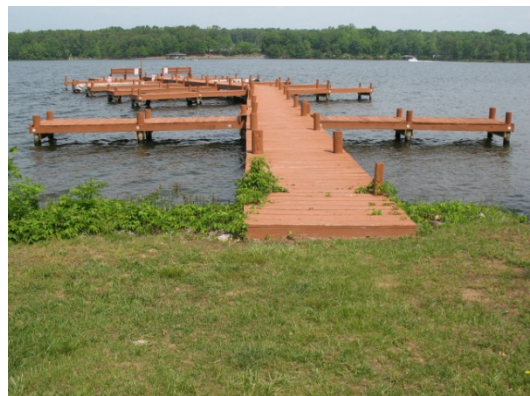
Overall view of wood boat dock
