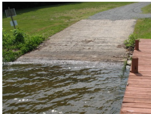
View of concrete boat ramp
