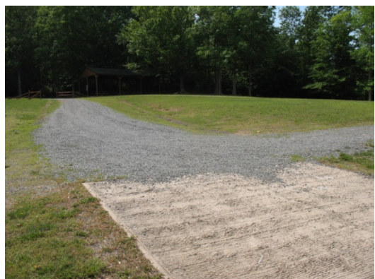
View of gravel road at boat ramp
