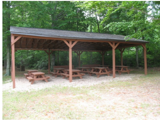
Side view of shelter
