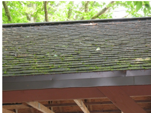
View of asphalt shingle roof with moss growth
