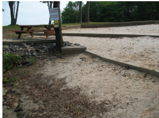
View of wood timbers at sand beach
