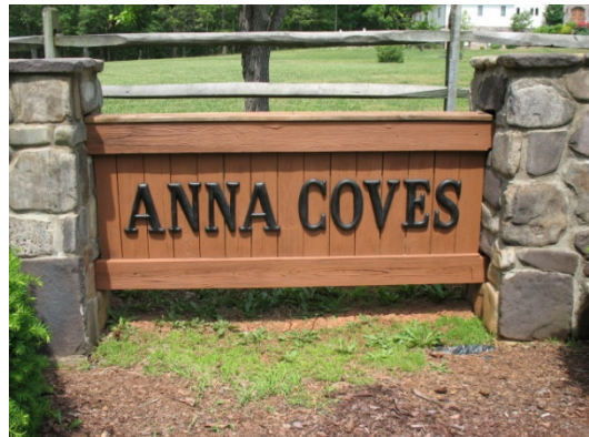
View of west side entrance monument wood frame and plastic letters
